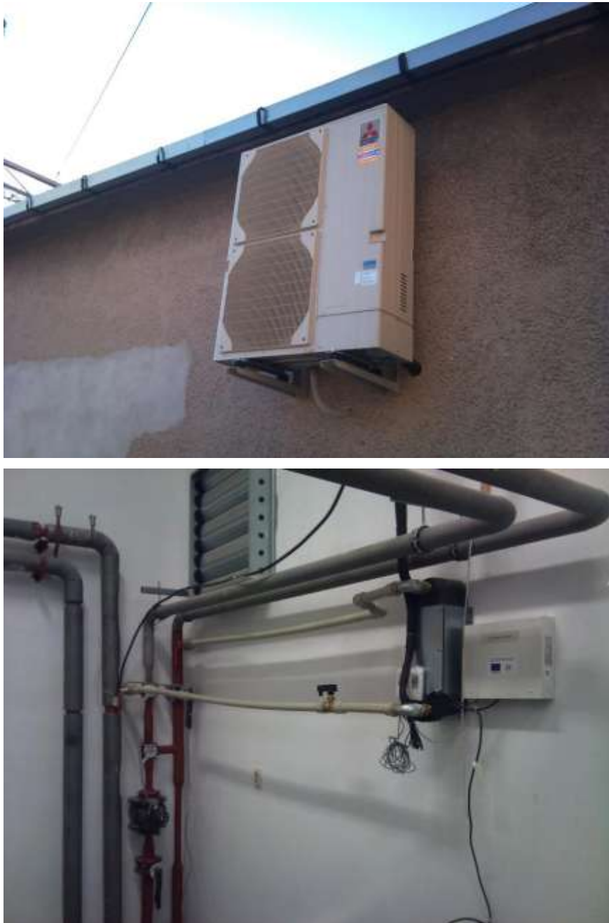
Fig.2 Electric heat pump „Zubadan“ and their accessory
