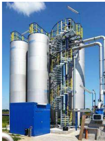
Figure 10: Moved- Biofiltration plus integrated sand- filtration
