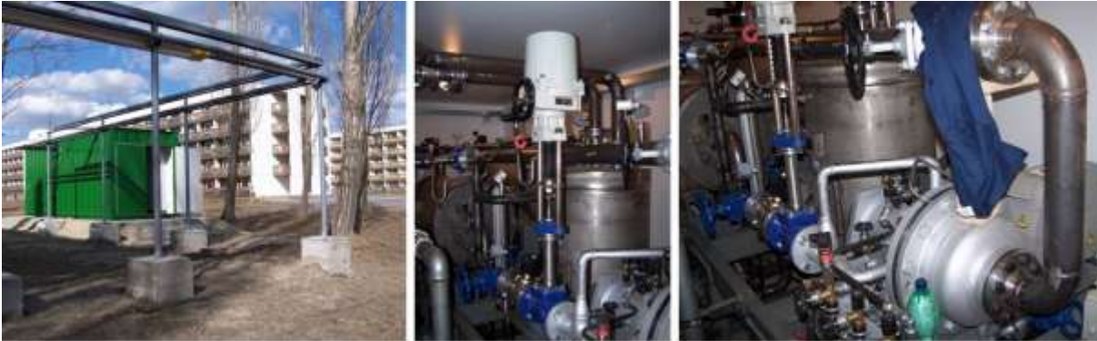
Fig. 3 Realized prototype with ORC
