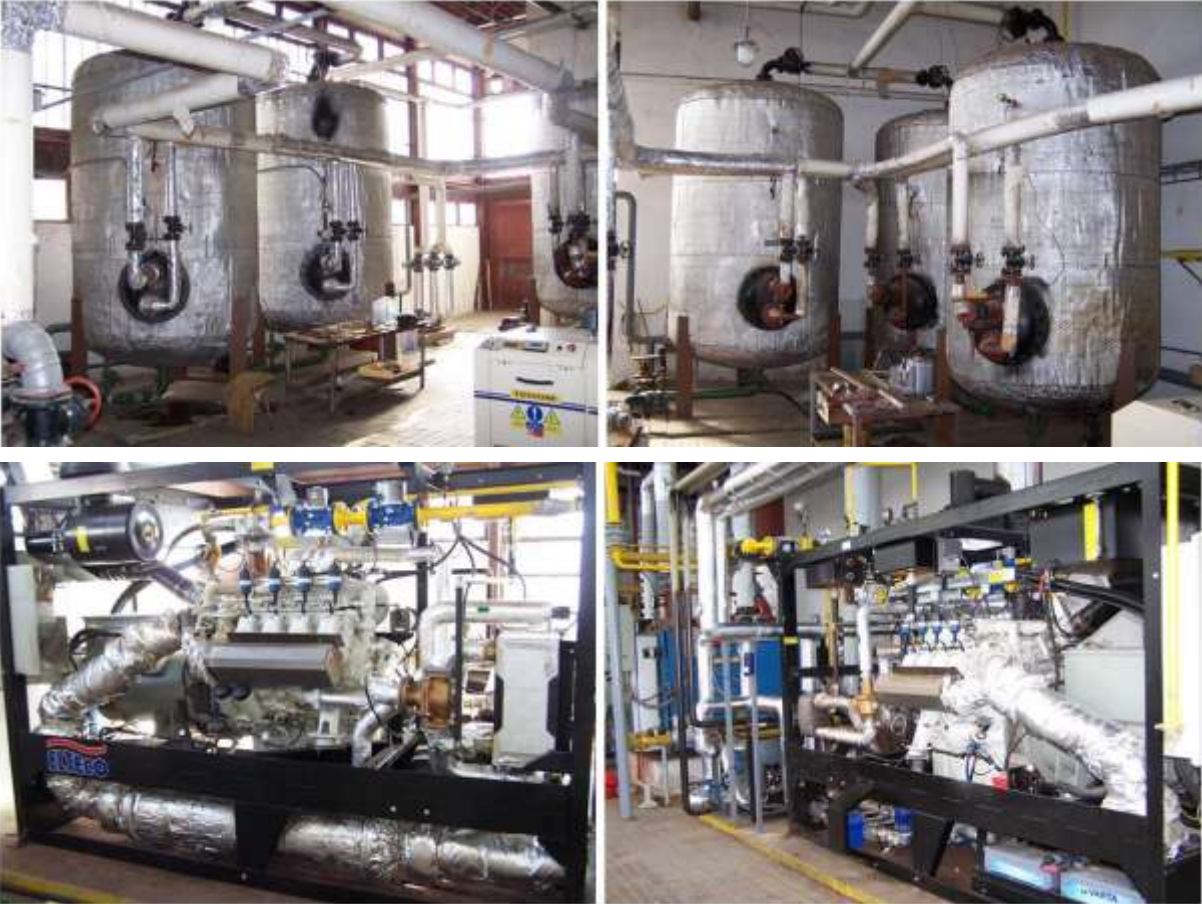
Fig. 2 Present cogeneration unit and hot-water tanks
